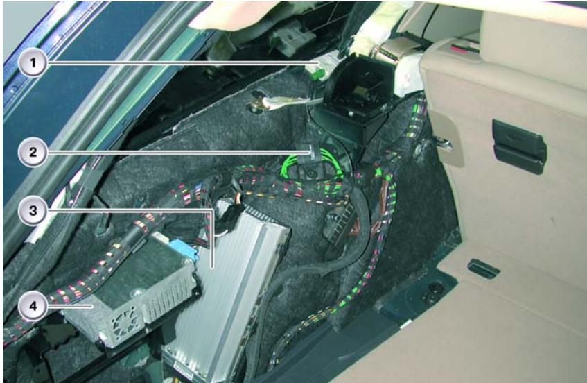
Control Units in Luggage Compartment, Left
